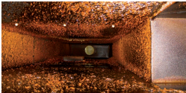
Typical grease buildup without AirMaid results in a high risk for dangerous duct fires and expensive cleaning bills.
