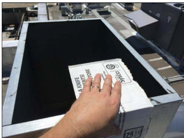
Cardboard test for grease at discharge
