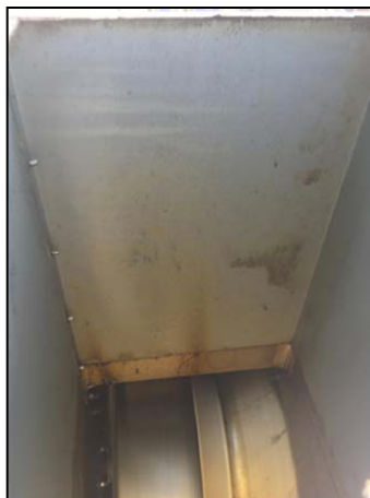
Looking down in exhaust stack at the fan wheel
