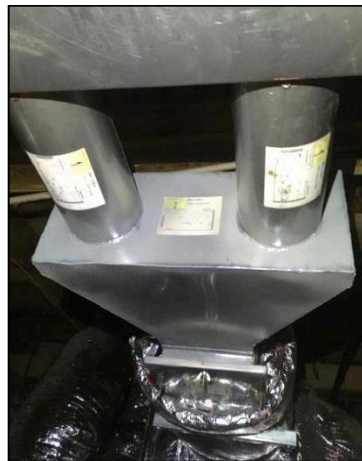
SS duct + access door + fd
