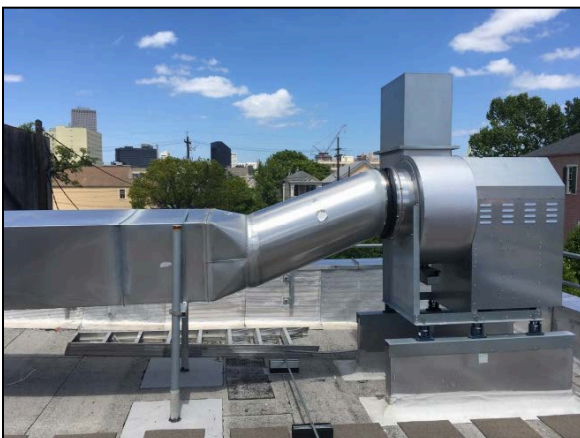
Kitchen exhaust fan on roof
