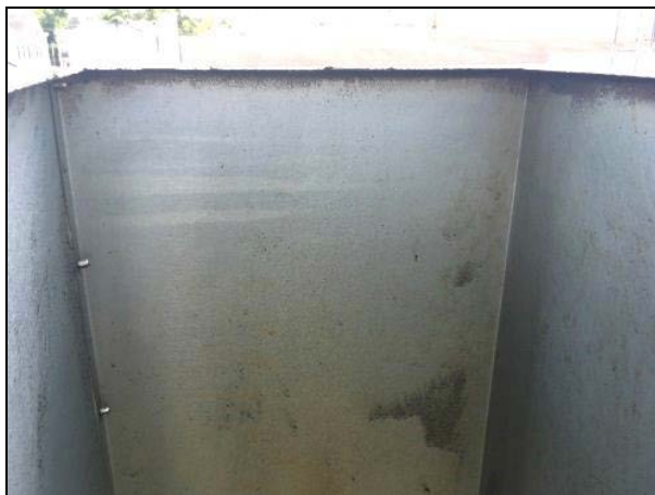
Inside kitchen exhaust stack
