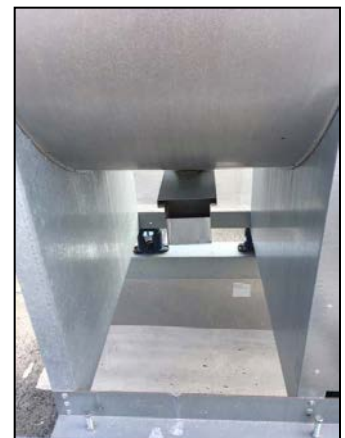
Grease trough location under the exhaust fan
