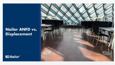
the idea for UFAD is to have a well-mixed lower level in the occupied space up to about 4.5 feet above the floor. From the thermocline at 4.5 feet to about 3 to 5 inches from the ceiling is a stratified space.
